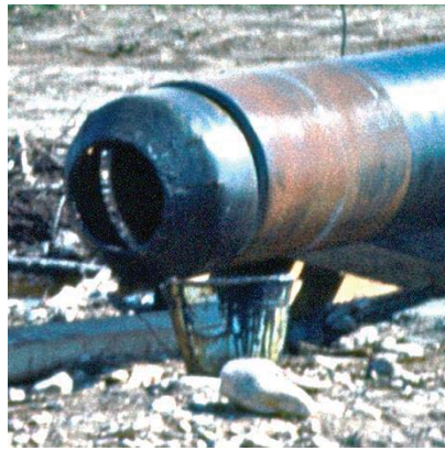
Figure 3. Detail Enlarged from Trugen Photo of Pipe Wrapping Machine Showing Wrapped Pipe (00010370012.tif)
