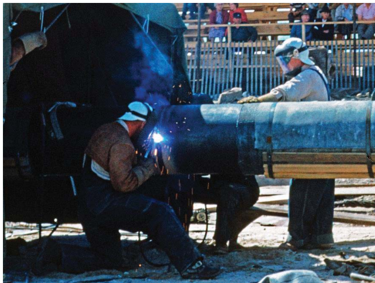
Figure 5. Trugen Photo of Pipe String Assembly Welding (00010370005.tif)
