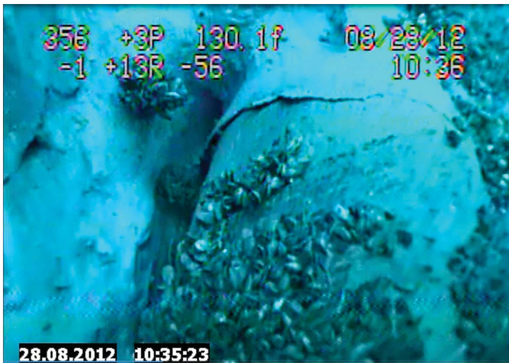
Figure 7. Photo Clipped from Enbridge 2012 Underwater Inspection Video of the East Line Taken on 8/28/2012 at 10:35:23 Showing Missing and Disbonded Coating
