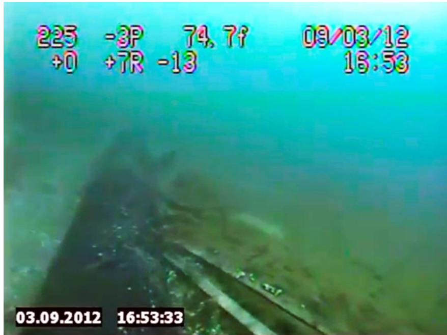
Figure 2. Frame Clipped from Enbridge Video Apparently Showing Detached Slats Because washouts caused by unforeseen currents in the Straits have left sections of the pipe unsupported in violation of seventy five foot requirement stated in the 1953 easement, Enbridge has been retrofitting the Straits Sections of Line 5 with modern, screw anchor supports. Enbridge Table 2. is a summary of these efforts.
