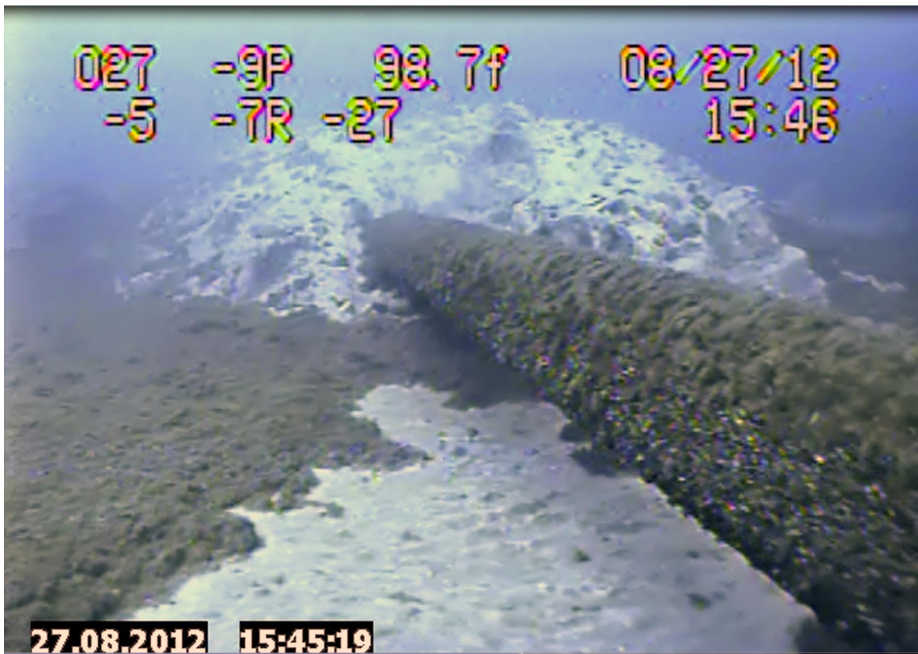
Figure 5. Typical Clay Fill Pile Placed in 1953 to Remediate an Unacceptably Long Unsupported span.
